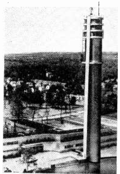
300-FOOT tower recently completed at the Federal Telecommunications Laboratories of the International Telephone and Telegraph Corporation at Nutley, N.J., U.S.A. It will be used for investigating U.S.W. propagation.
